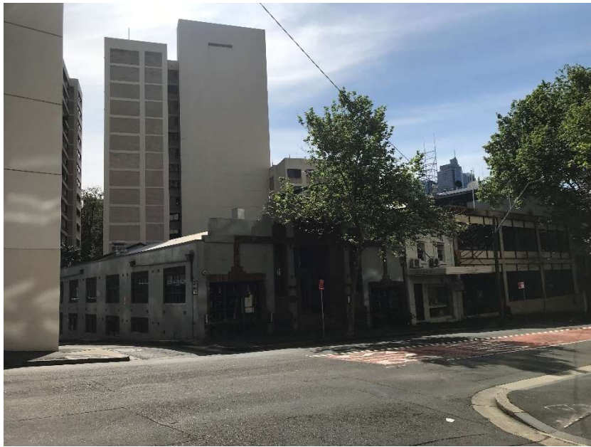
Figure 46: 55-61 Riley Street – former garage, Woolloomooloo. The subject site can be seen further to the right.
