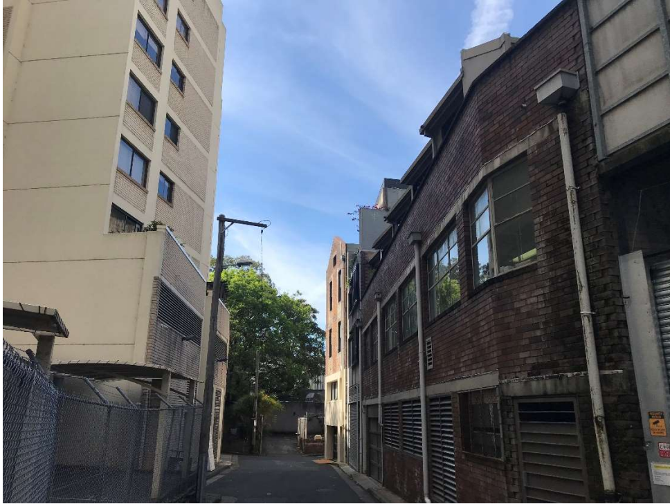
Figure 40 - Rear view of 51 Riley Street from Busby Lane. Note the proximity of the multi storey residential building immediately behind the subject site.
