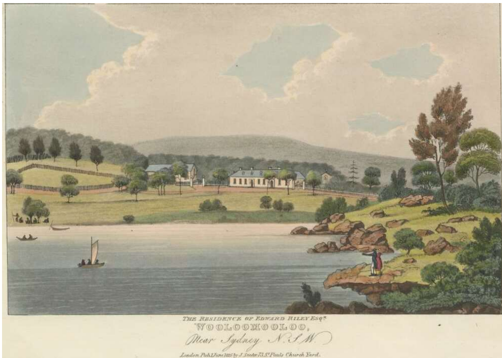
Figure 6: The residence of Edward Riley, Esq., Woolloomooloo [Woolloomooloo] near Sydney, NSW, Joseph Lycett, 1825 (Source: National Library of Australia, PIC Volume 68 #U452 NK2707/5)
