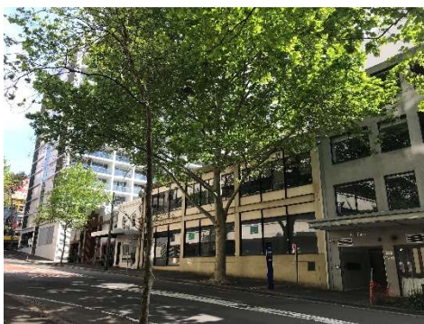
Figure 35 - 51 Riley Street (centre of image)
